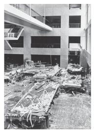
FIGURE 9-1 Elevated walkway collapse in a Kansas City hotel in 1981. How a simple physics calculation could have prevented the tragic loss of over 100 lives is considered in Example 9–12.
