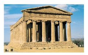
FIGURE 9-21 This Greek temple, in Agrigento, Sicily, built 2500 years ago, shows the post-and-beam construction. The columns are under compression.
