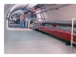
FIGURE 32-3 The interior of the tunnel of the main accelerator at Fermilab, showing (red) the ring of superconducting magnets used to keep particles moving in a circular path at the 1-TeV Tevatron.
